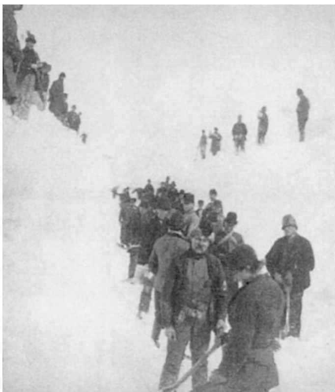
Fig. 2 Cleaning snow away from the railroad tracks at Kelly's Cut, 0.8 km (0.5 miles) west of Sleepy Eye, Minnesota, in March 1881. Image courtesy of Chicago and North Western Archives
